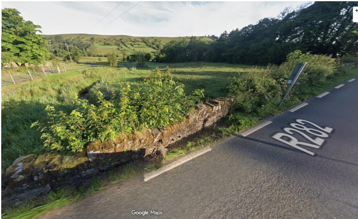
Figure 2- photo at point where water course passes under the bridge on R282 flowing towards Ballagh River.
